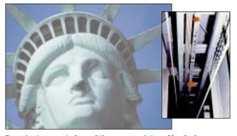
The service elevator on the Statue of Liberty uses a vertical run of Four-Bar for power. Important features are reliability and compactness for this 245 foot high run.
