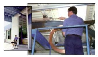
The Tri-Bar and Four-Bar conductors are supplied in coils, and inserted in the housing slots from one end of the run. Long runs are coiled on a cross for added stability and to use with payoff stands.
