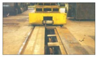
This trench-mounted Tri-Bar withstands dirt, oil and moisture to electrify a steel coil transfer car.
