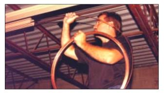
The key to superior performance is eliminating joints in the conductors. The copper conductors come in coils, as shown, and are slid into the housing from one end of the conductor system.
