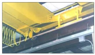
The Four-Bar provides continuous copper bars, joint-free for the entire runway length. Four conductors take up only 2 5/8 inch of horizontal space.
