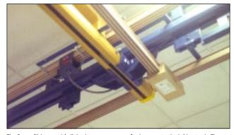
The Power Pickup on this light duty crane runway feeds power to the bridge track. The drag on the manually pulled hoist is negligible.
