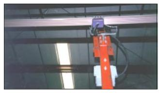
Four-Bar replaced the festoon systems on four transfer car runways in this plant, as well as additional runs in a second plant. Owners are happy with the trouble-free performance
