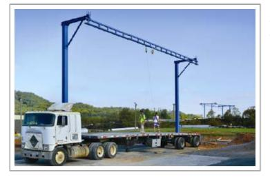
They found a solution, with a lower cost than a new building and allowed the workers to remain on the truck, in the form of two free standing Tether Track fall protection systems by Gorbel. The primary system features two cantilevered monorails, which enables two flatbeds to be loaded in the same area simultaneously. Each monorail uses Gorbel's dual track, allowing two workers to pass one another safely without disconnecting the lanyard from their harness. A second Tether Track system
